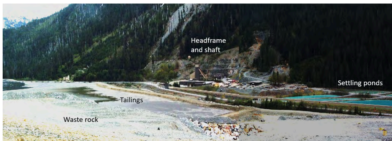
Figure 2.4.5: The tailings pond at the Myra Falls Mine on Vancouver Island. The dry rock in the middle of the image is waste rock. Myra Creek flows between the tailings pond and the headframe. The settling ponds (right) are used for processing water from the concentrator.
